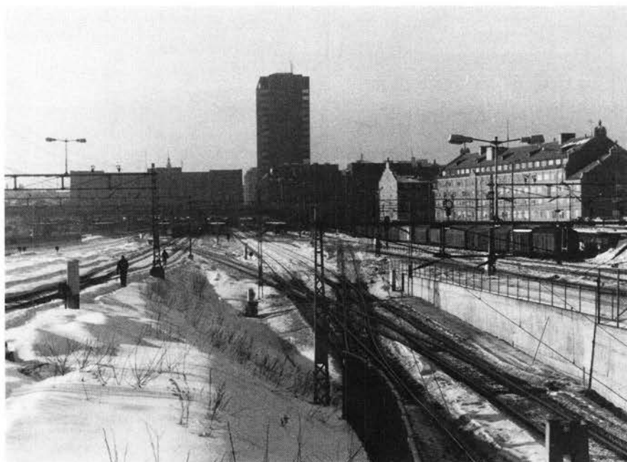
Oppkjøring fra tunnelen under Brynsbakken inn mot Oslo S. Track connection from the tunnel under Brynsbakken towards The Central Station.
