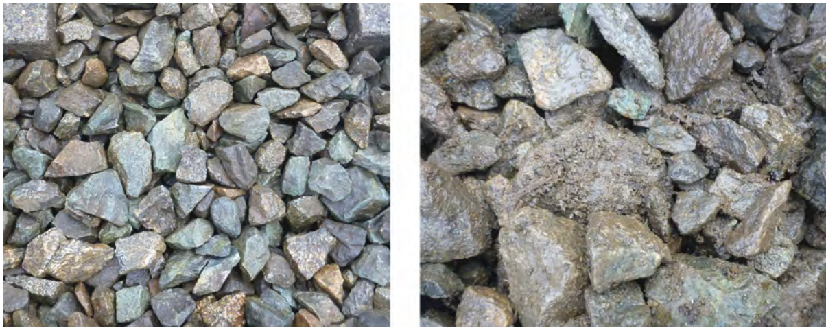
Figure 26: Left: Surface ballast quality. Right: Lightly fouled ballast sample excavated from the same site.
