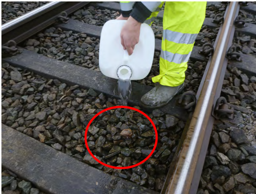
Figure 27: Water being poured into the ballast at the first test site, marked in red.
