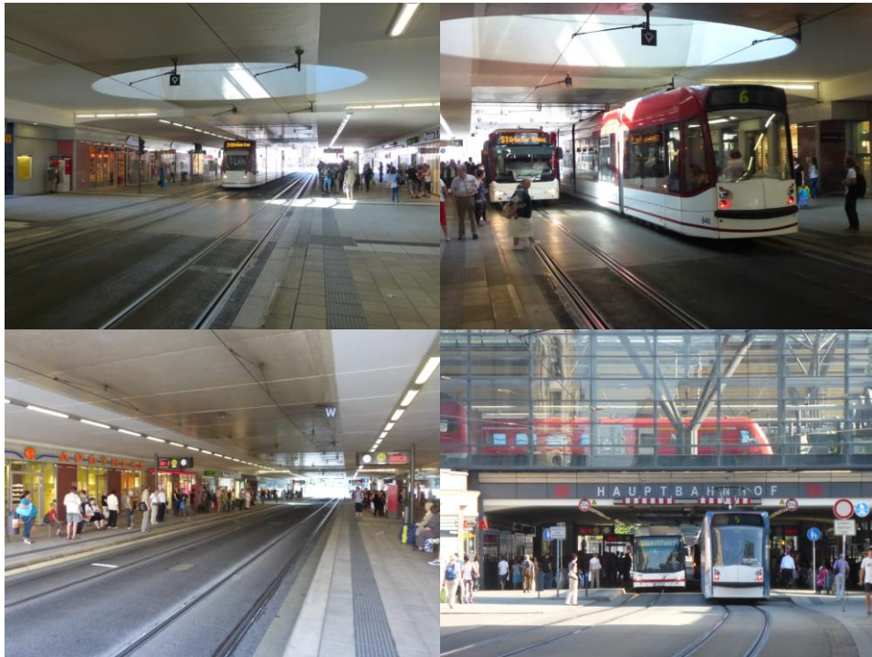
Erfurt: main railway station interchange for trams and buses
