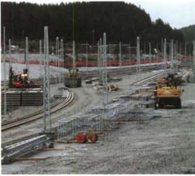
Ganddal freight terminal is under construction. Photo: Kjell Bakken
