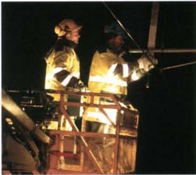
Overnight work on the overhead lines. Photo: Øystein Grue
