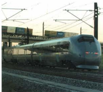
The Oslo–Eidsvoll main line crosses the Gardermoen airport line. Photo: Øystein Grue
