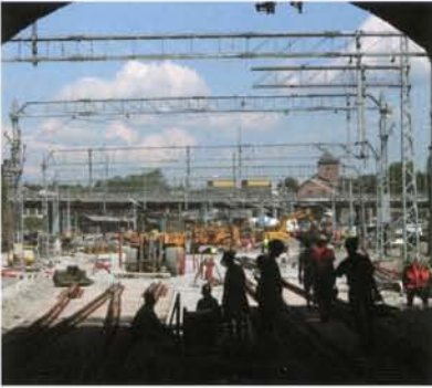
Construction work at Asker station, summer 2005. Photo: Olaf Bjerknes
