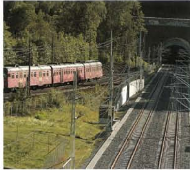
The old and new double tracks side by side at Solstad, Asker. Photo: Øystein Grue
