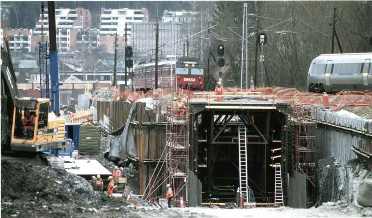
Construction works at Jong. (Photo: Rune Fossum)
