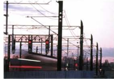
Gardermoen airport line
