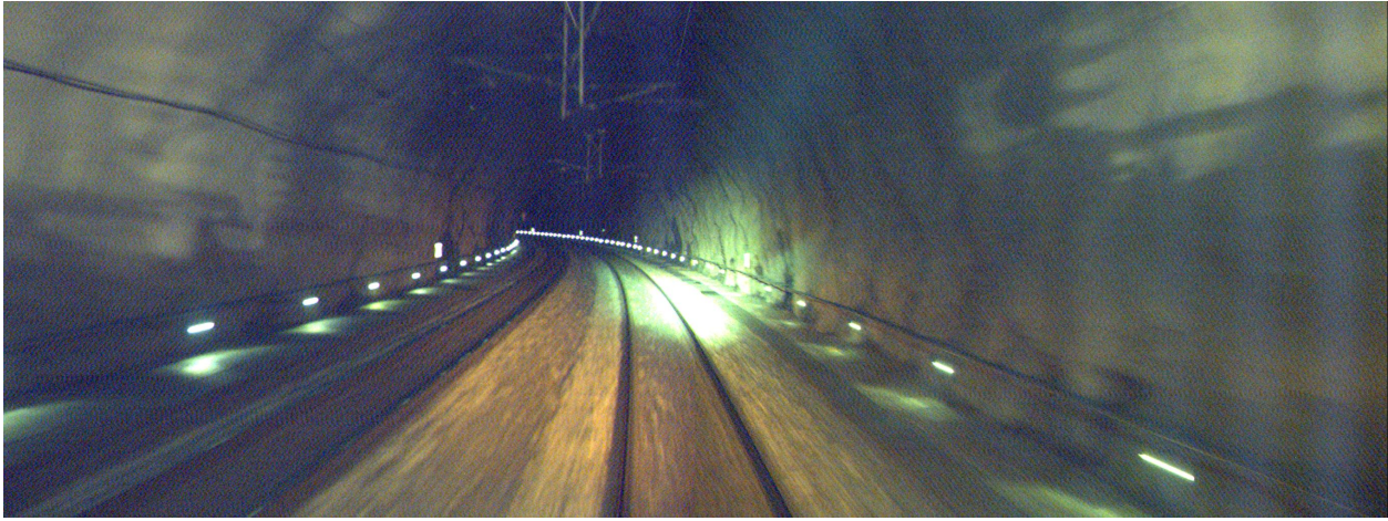
Figure A.3: Tanumtunnelen at 16.492 km
