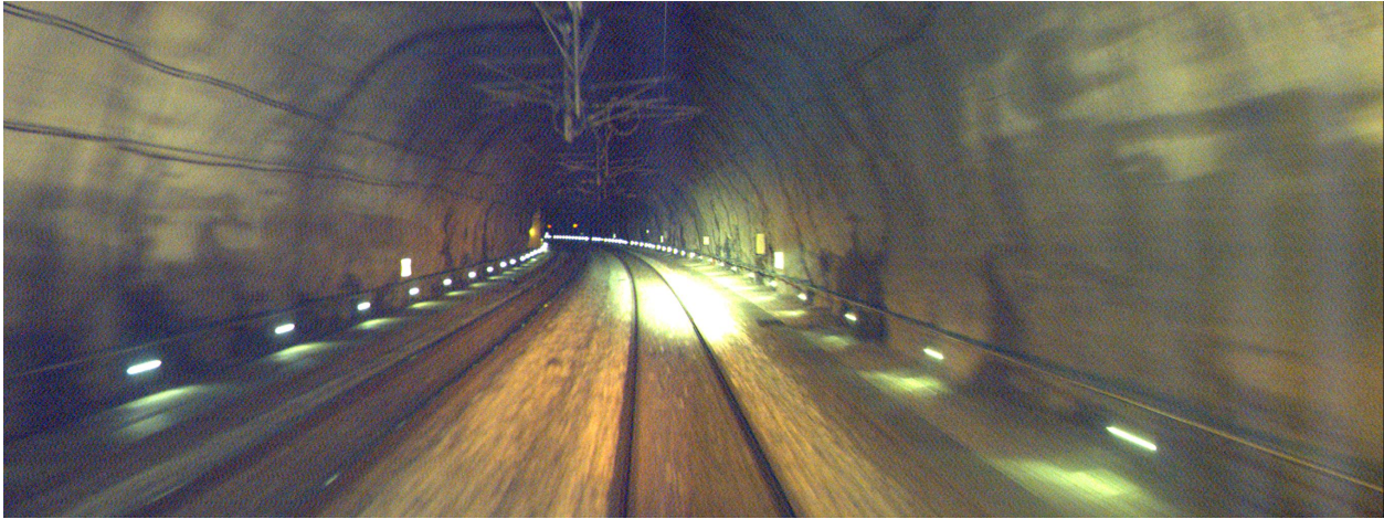
Figure A.4: Skaugumtunnelen at 19.591 km
