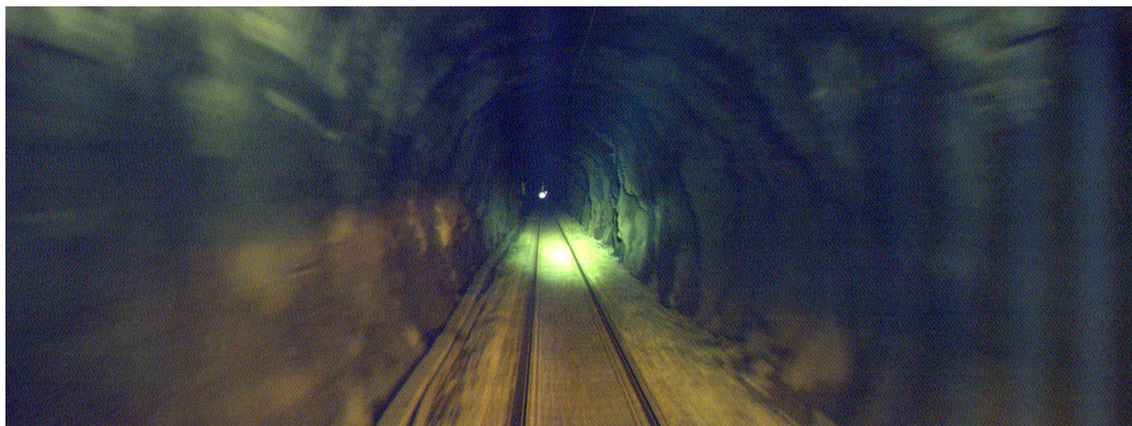
Figure A.10: Tronåstunnelen at 470.747 km
