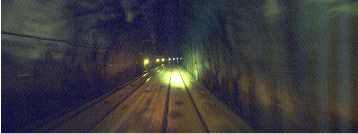
Figure A.5: Lieråsentunnelen at 37.038 km
