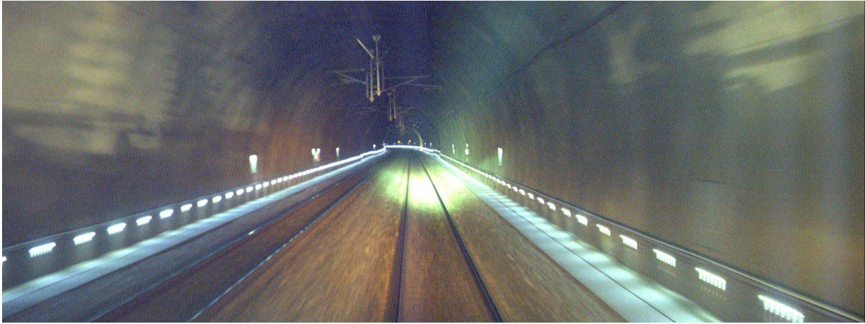
Figure A.2: Bærumstunnelen at 8.092 km
