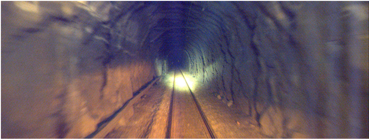
Figure A.6: Siratunnelen at 462.047 km
