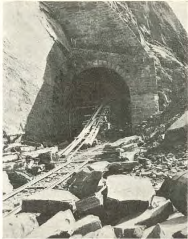
Fig. 11. Utmuring. Kleivene tunnel.
