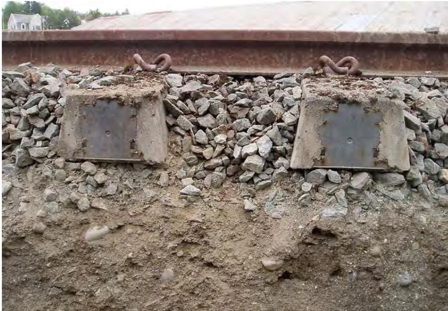
**Figure 1.3. Fouled ballast on Stavne-Leangen Line near Trondheim.**
