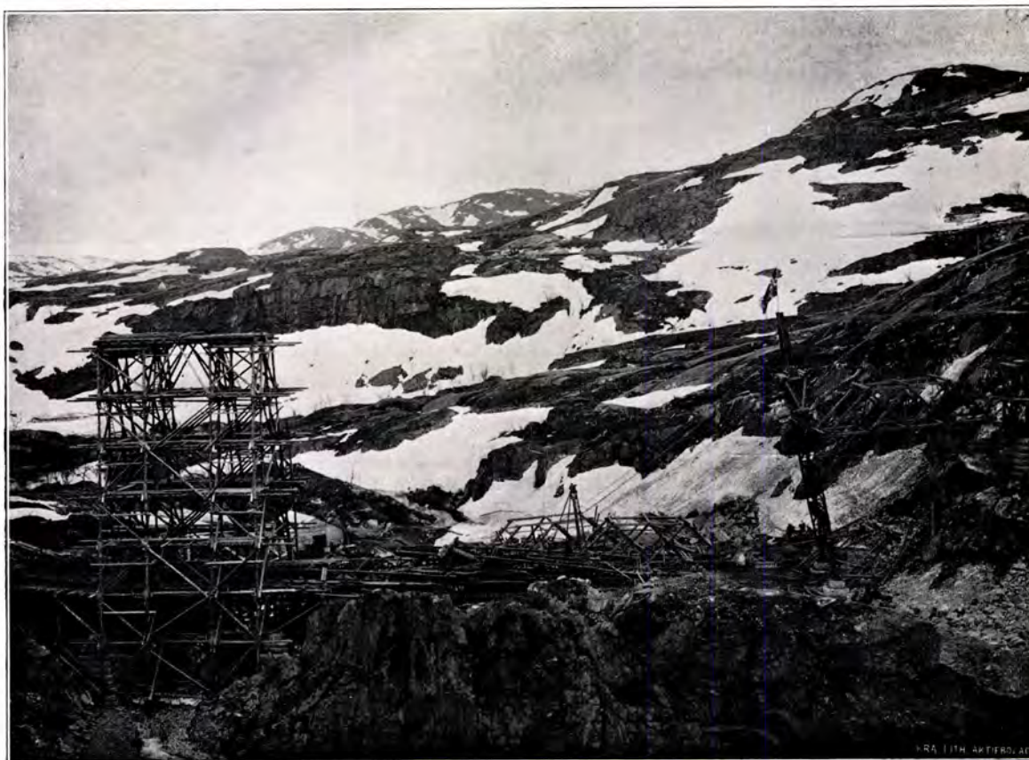
BRO OVER NORDDALSENDEN UNDER MONTERING.
