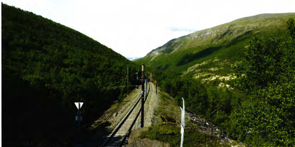
Figure 18. Existing railway line near Kongsvoll Station.
