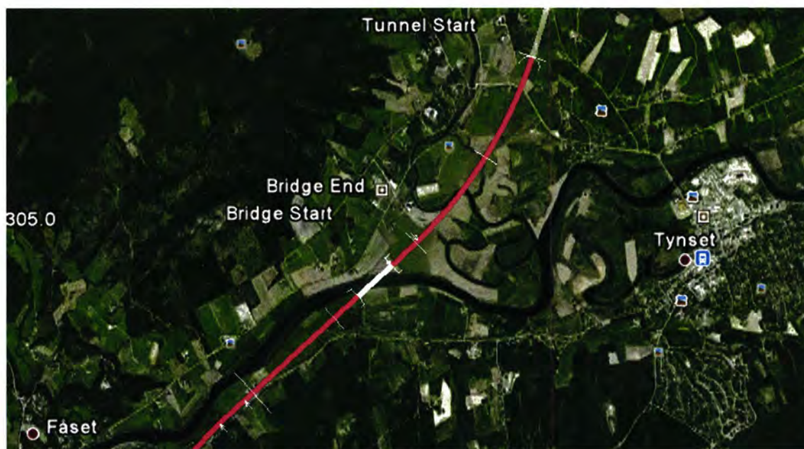
Figure 163. Bridges crossing river Glomma close to Tynset. The flooding situation will possibly require bridge viaducts adjacent to the bridge.
