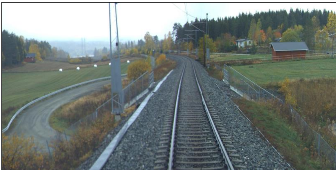
Figure 3.8 - ROGER 1000 photo showing the transition zone a few meters before the culvert (Source: Bane NOR)
