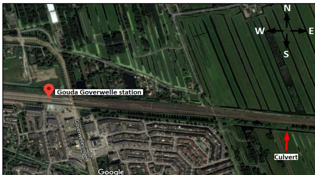
Figure 1.1 – The Utrecht-Gouda railway line and location of the stiff square concrete culvert (Source: Google maps)
