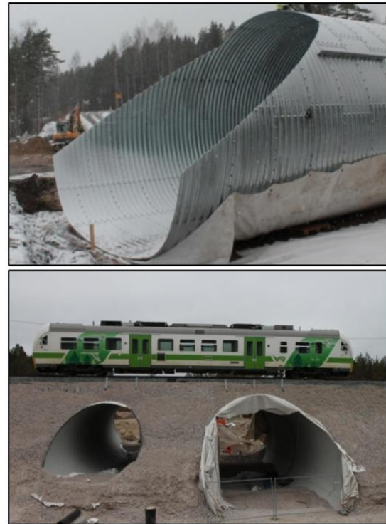
Figure 4.26 – The «Torppari» culvert underpasses at Hank-Karjaa line (Modified after Asp, O, 2014)
