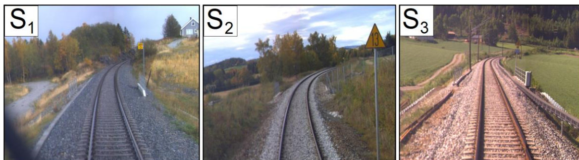
Figure 5.3 – ROGER 1000 photos at the site conditions at S 1 ) Sjånes, S 2 ) Holme and S 3 ) Viker culvert
