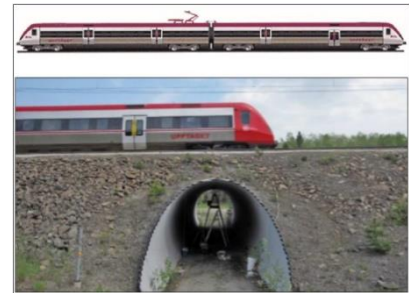
Figure 4.24 – The «Rörbru i Märsta» culvert during a X-52 train passage at 170 km/h (Modified after Andersson. Et. al, 2012)
