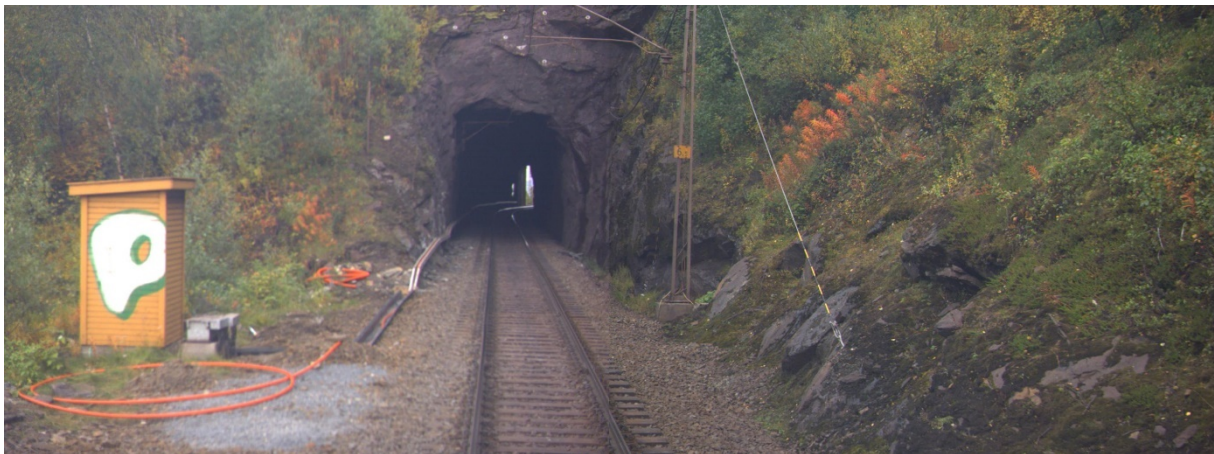
Figure 4-13 Ofoibanen km 6,47 (Bane NOR, 2017)
