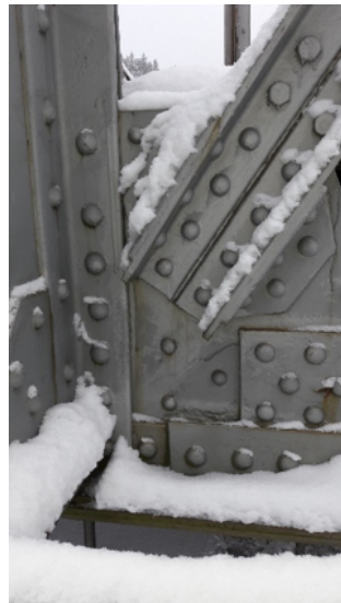
Figure 5.7: A typical plated connection on the Hell bridge
