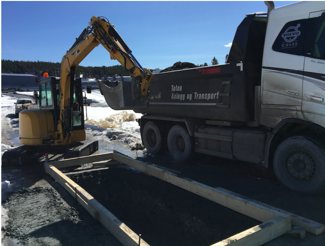
Figure 3.16 – Excavation of test pit
