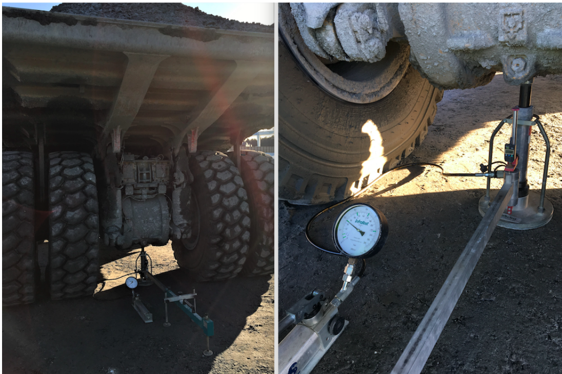
Figure 3.12 – Plate load test equipment rigged for testing at Åsland deposit site
