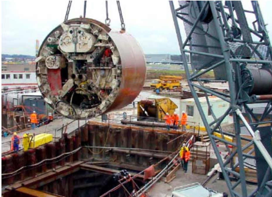
Figure 32: Installation of a hydro shield TBM for tunneling under Zurich airport (Amberg archive)
