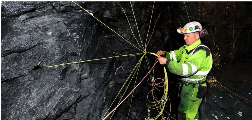
Figur 2: Lading for salvesprengning
