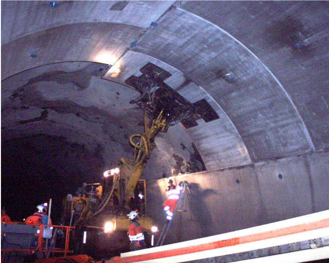
Figur 15: Betong elementhvelv under montering
