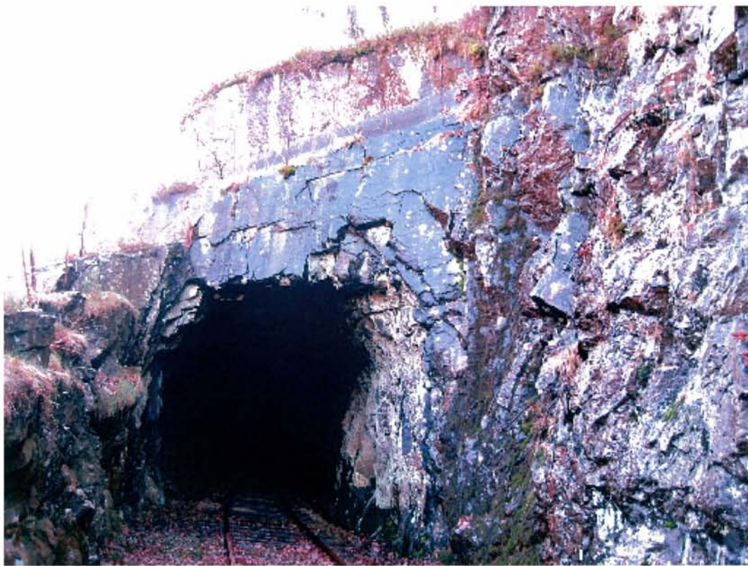
Km 12,960 12 Nov 2008 kl 11:40 Loga tunnel N
