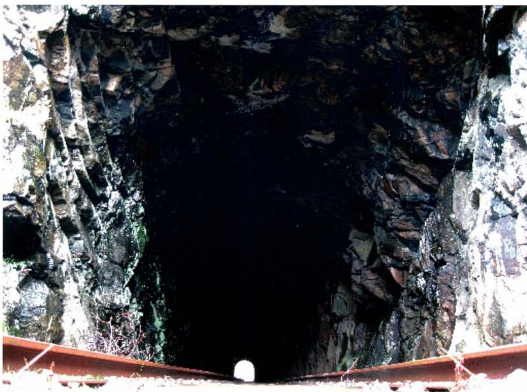
Km 15,830 11 Nov 2008 kl 14:18 Kraketo tunnel N
