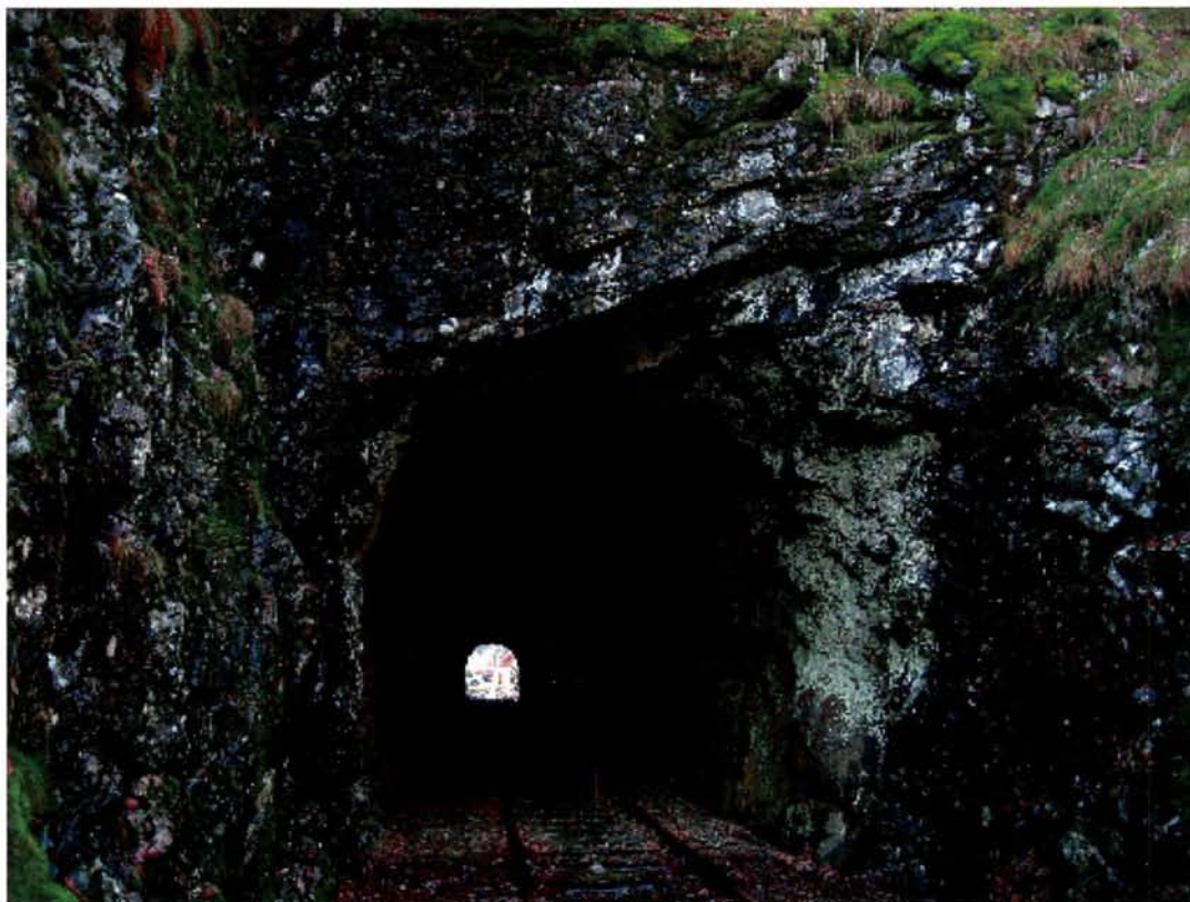
Km 11,230 12 Nov 2008 kl 14:46 Soland tunnel II N
