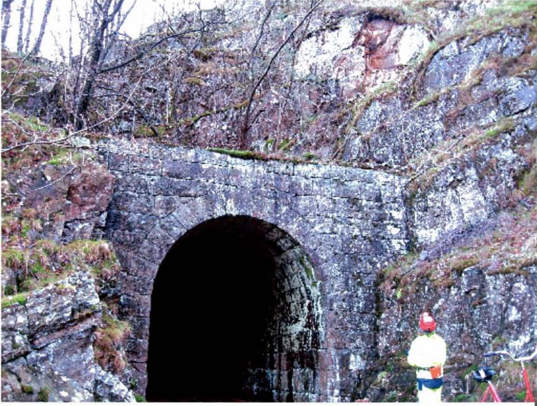
Km 11,950 12 Nov 2008 kl 13:28 Stromland tunnel N
