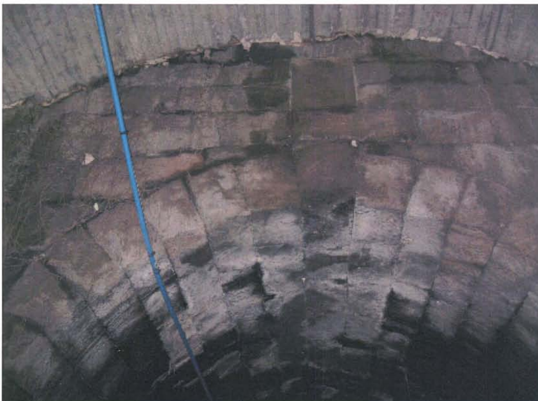
Km 16,990 11 Nov 2008 kl 9:28 Trolldal tunnel S
