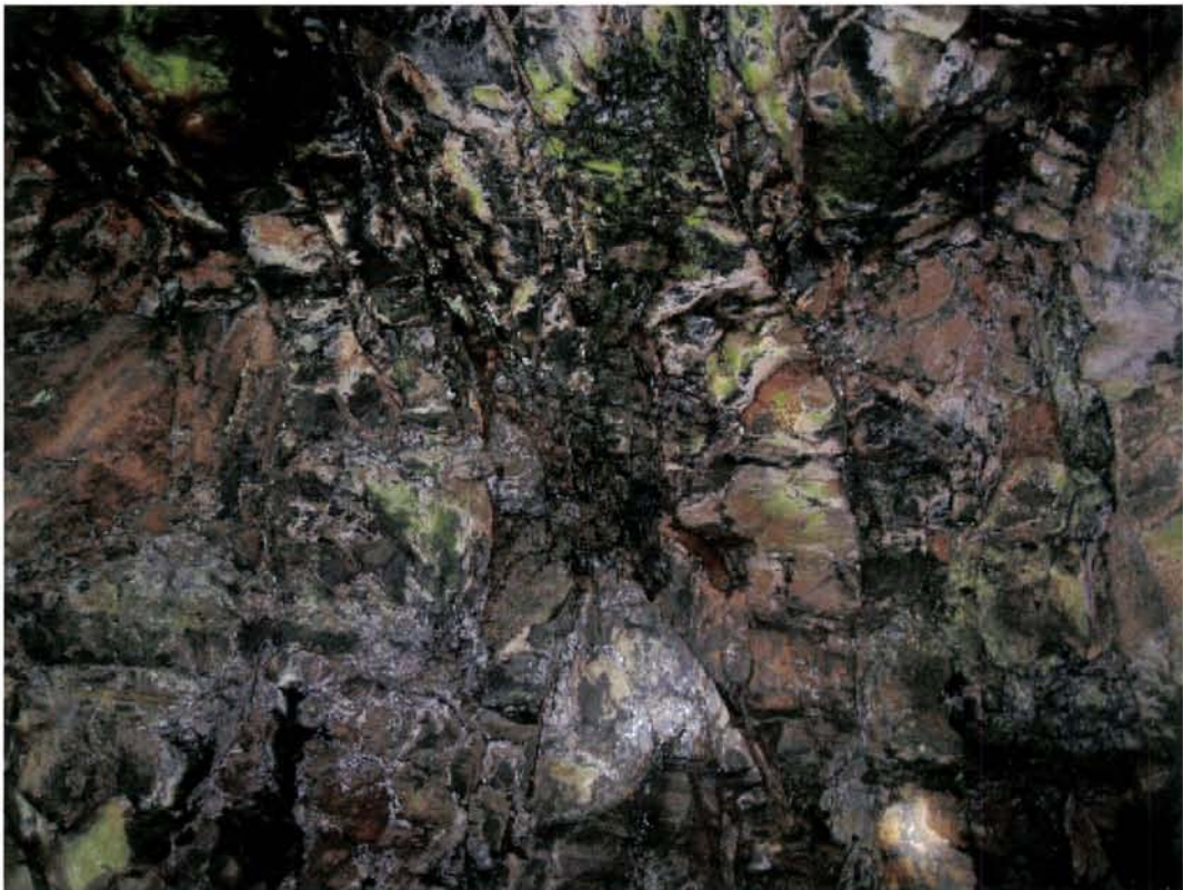
Km 12,135 12 Nov 2008 kl 13:15 Stromland tunnel S
