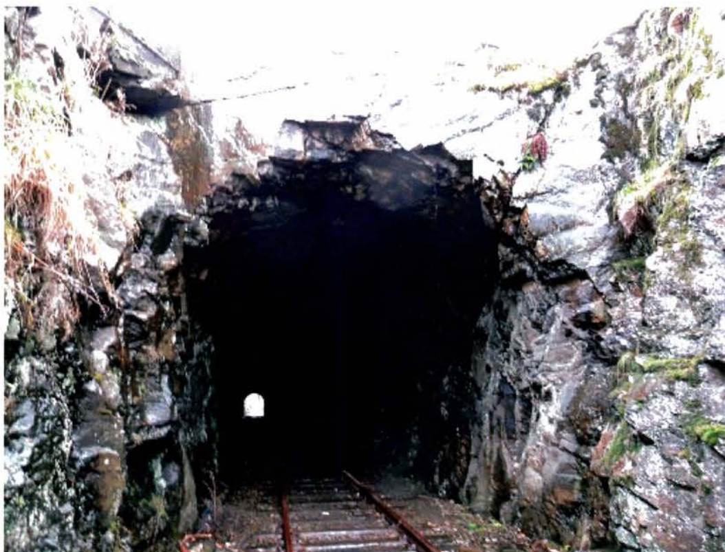
Km 15,830 11 Nov 2008 kl 14:17 Kraketo tunnel N
