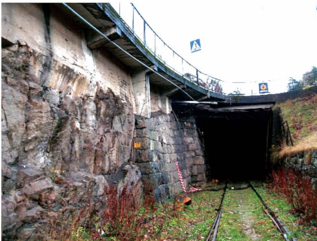
Km 16,990 11 Nov 2008 kl 9:10 Trolldal tunnel S
