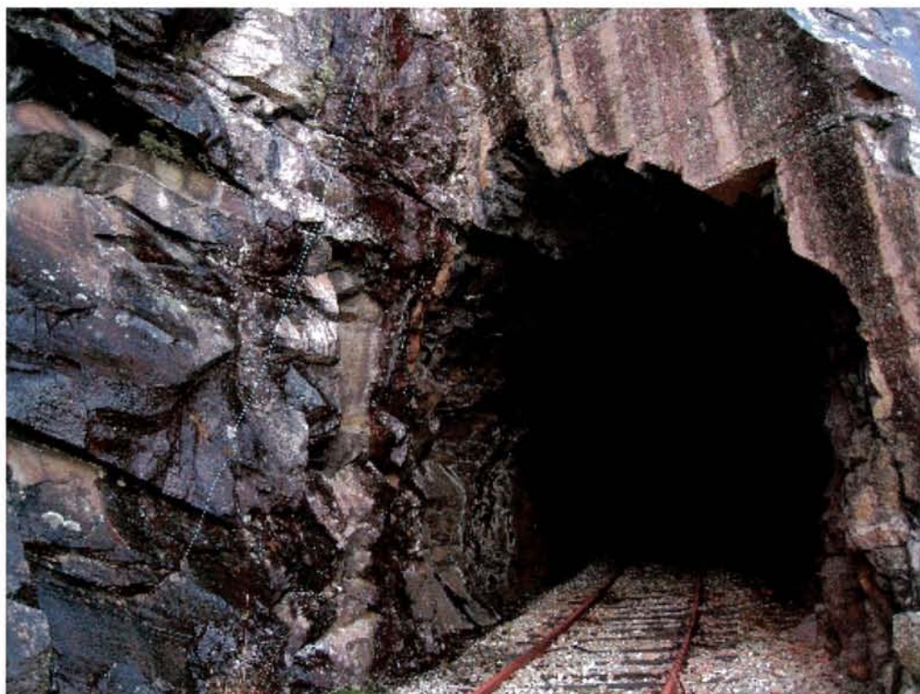
Km 10,540 12 Nov 2008 kl 15:23 Loia tunnel II S
