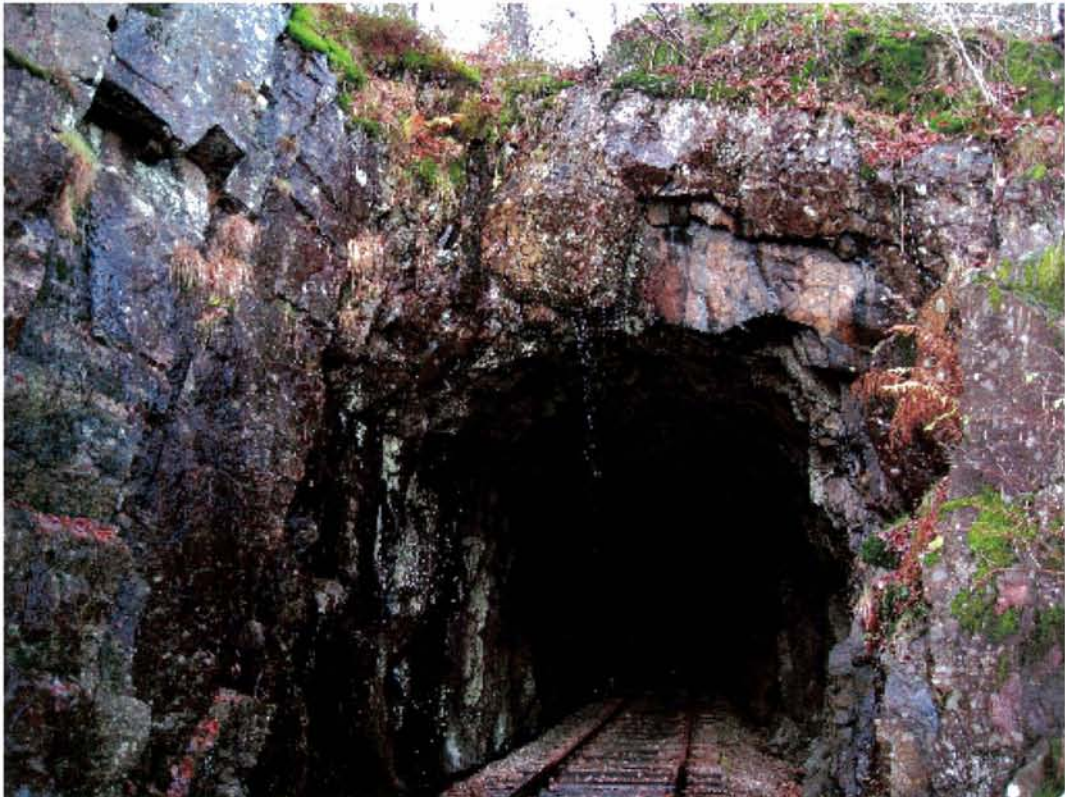
Km 12,135 12 Nov 2008 kl 13:09 Stromland Tunnel S
