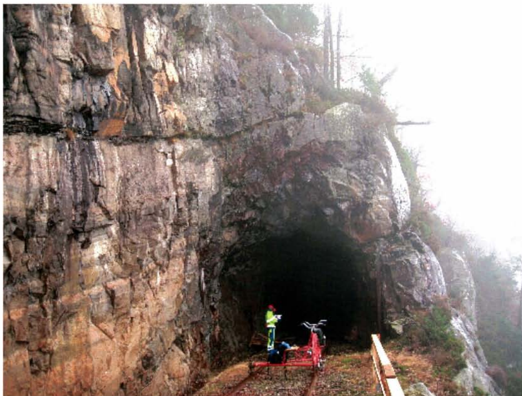
Km 4,520 13 Nov 2008 kl 11:58 Migaren tunnel N
