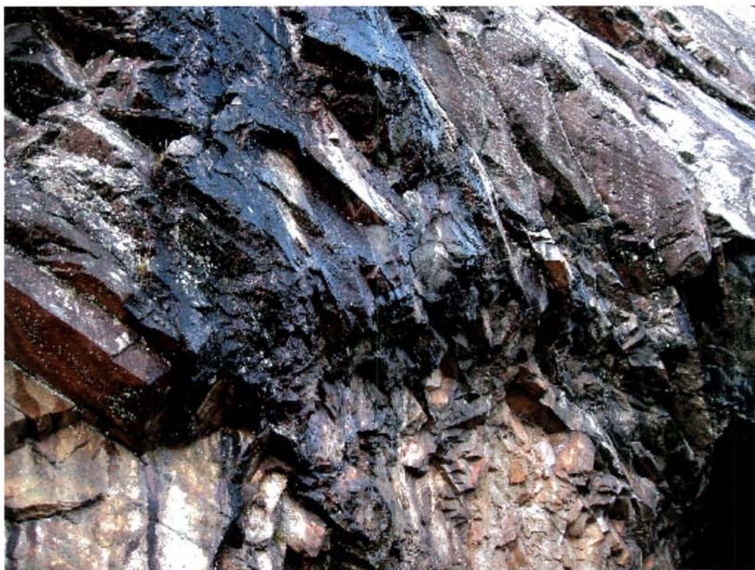
Km 10,897 12 Nov 2008 kl 15:09 Loia tunnel | S
