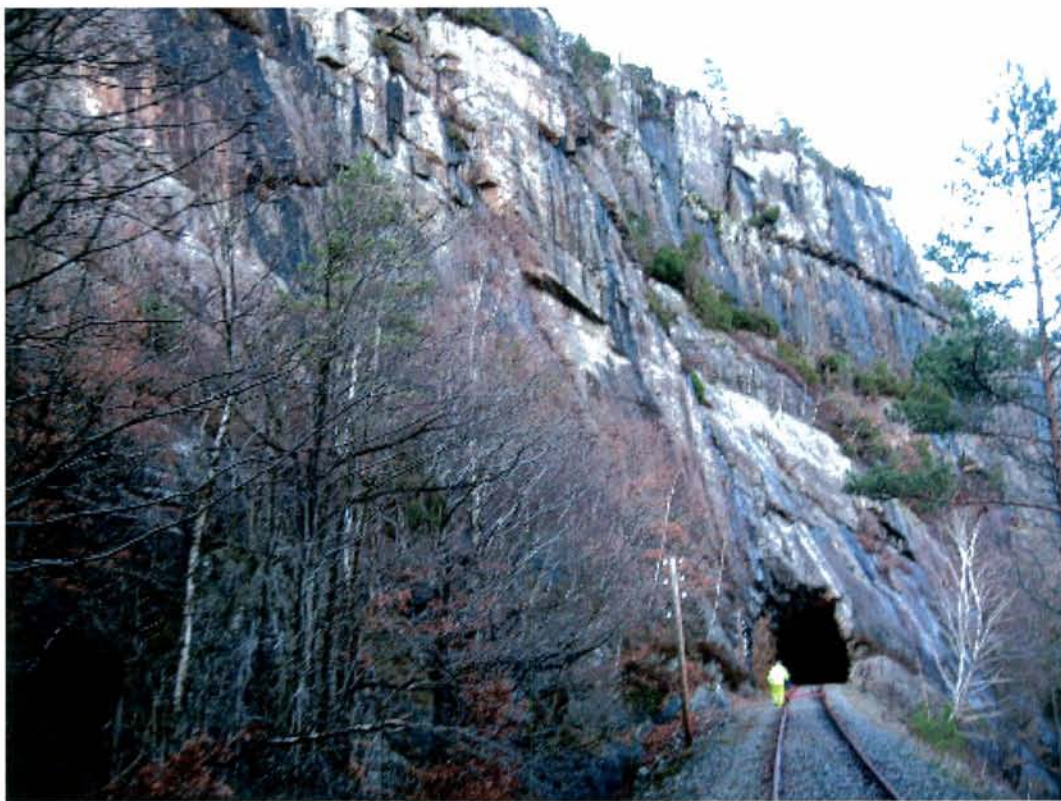
Km 10,897 12 Nov 2008 kl 15:04 Loia tunnel | S
