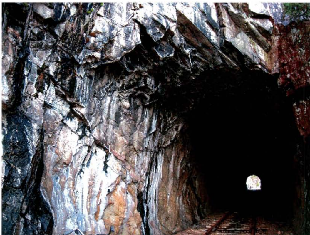
Km 11,335 12 Nov 2008 kl 14:36 Soland tunnel II S
