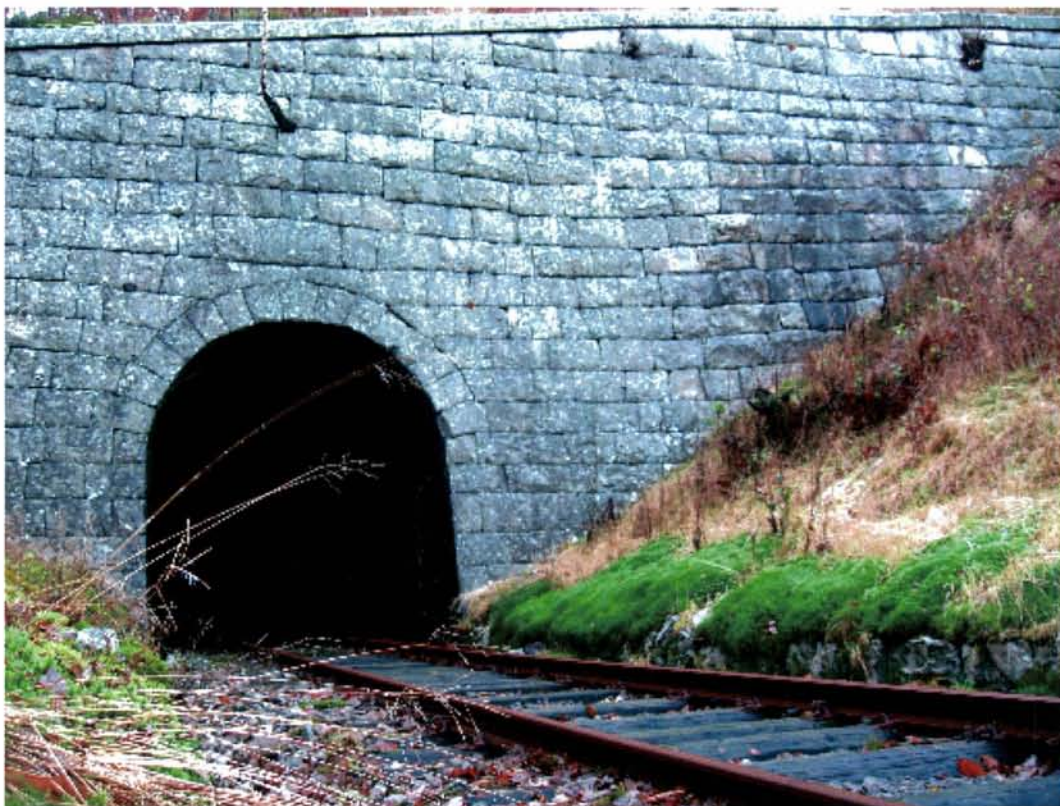
Km 9,563 12 Nov 2008 kl 15:56 Lavold Tunnel S
