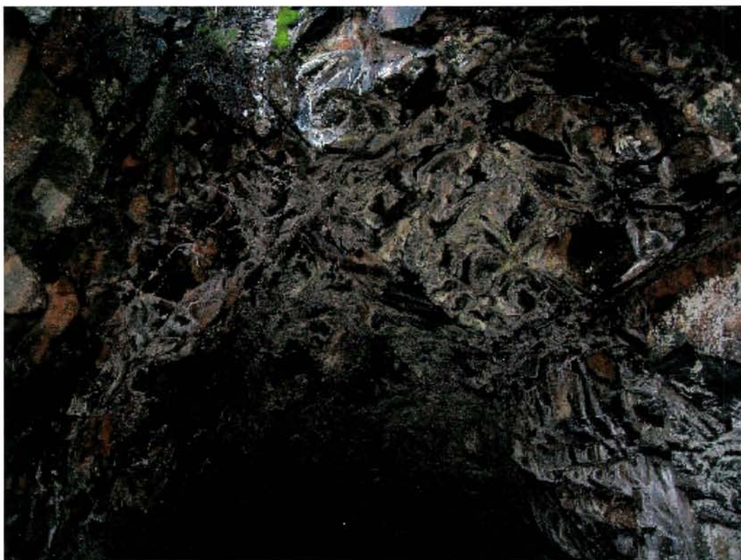
Km 10,430 12 Nov 2008 kl 15:34 Loia tunnel II N
