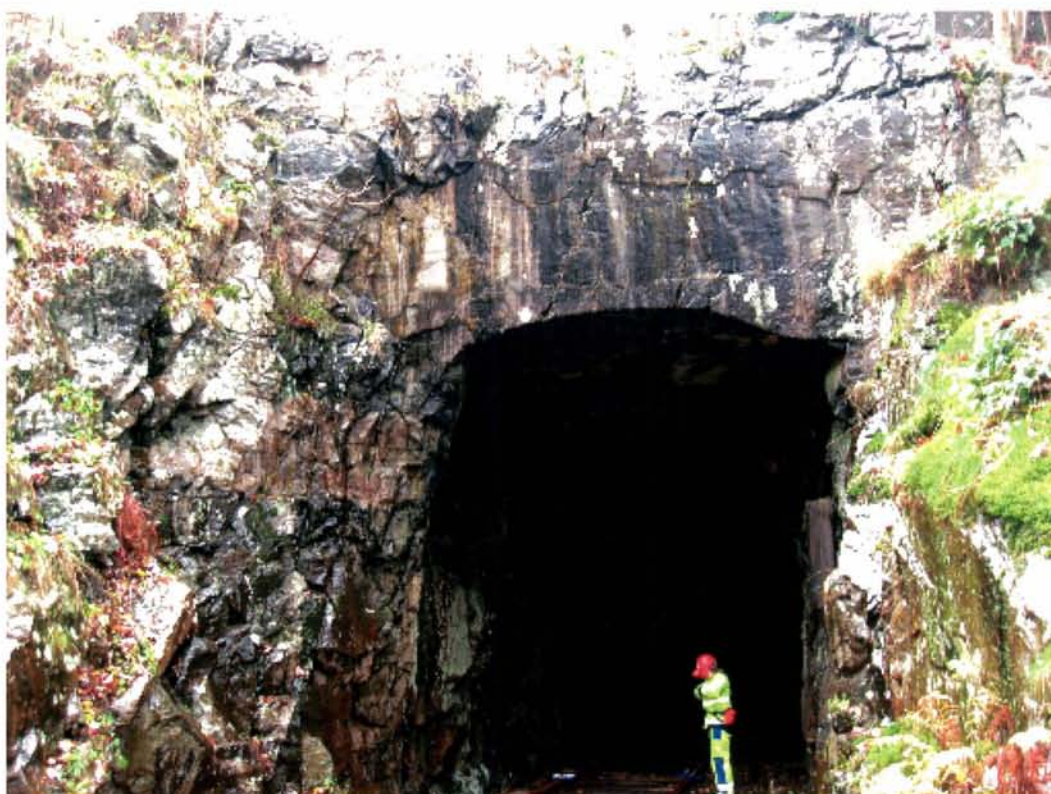
Km 16,090 11 Nov 2008 kl 12:09 Auestad tunnel N
