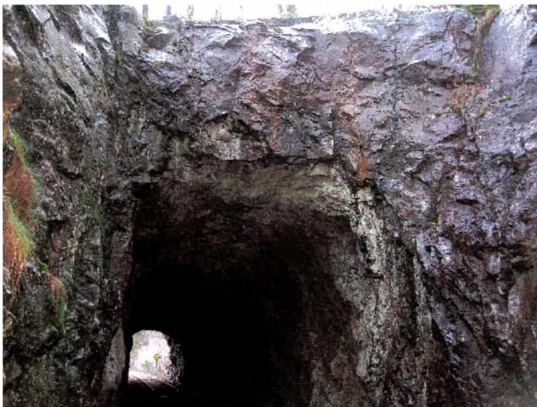
Km 11,030 12 Nov 2008 kl 15:01 Soland tunnel III N
