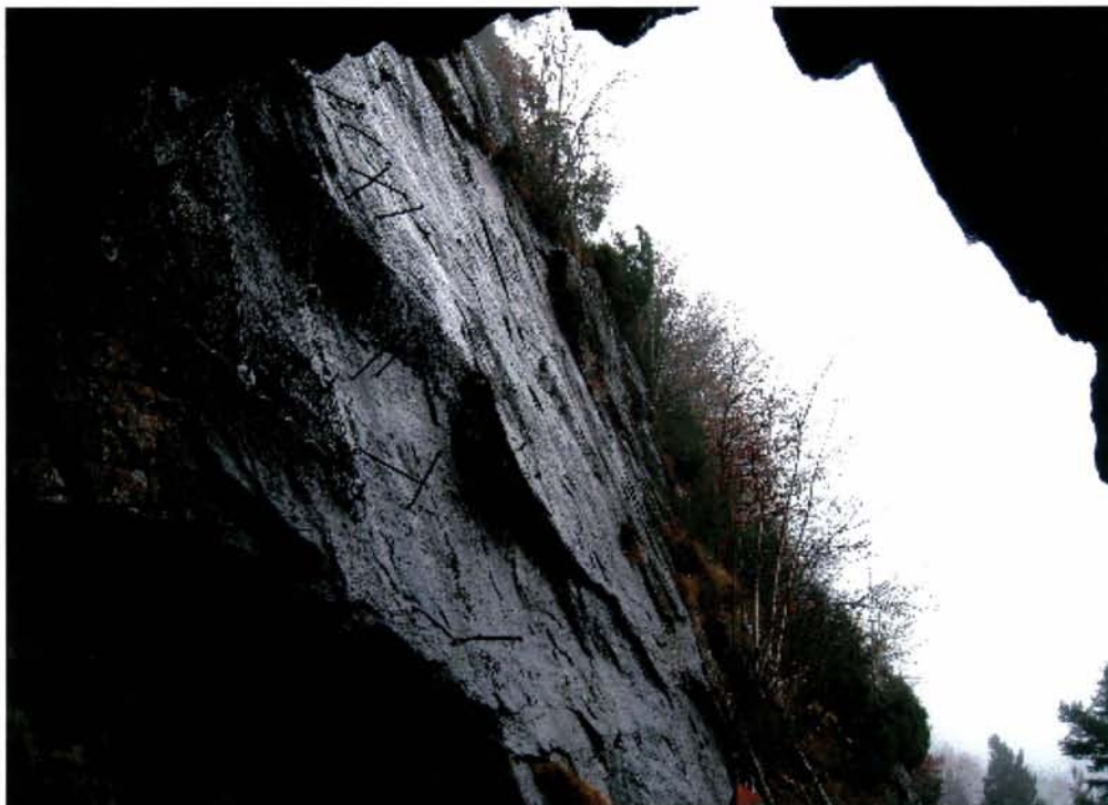
Km 5,185 13 Nov 2008 kl 11:45 Migaren tunnel S
