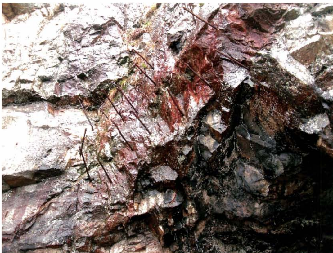
Km 4,520 13 Nov 2008 kl 12:00 Migaren tunnel N
