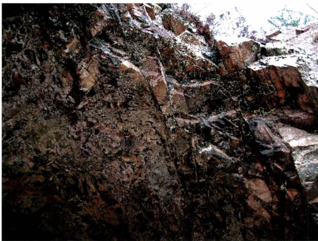
Km 11,081 12 Nov 2008 kl 14:54 Soland tunnel III S
