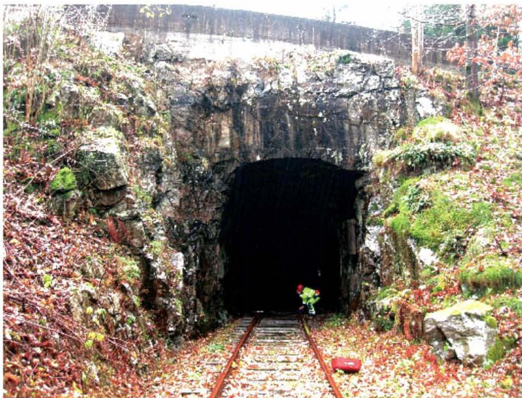
Km 16,090 11 Nov 2008 kl 12:08 Auestad tunnel N
