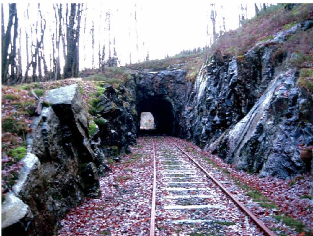
Km 11,030 12 Nov 2008 kl 15:03 Soland tunnel III N
