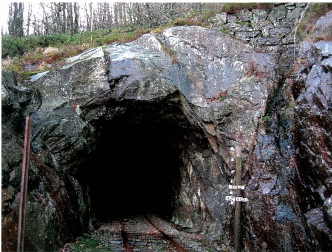
Km 10,580 12 Nov 2008 kl 15:17 Loia tunnel I N
