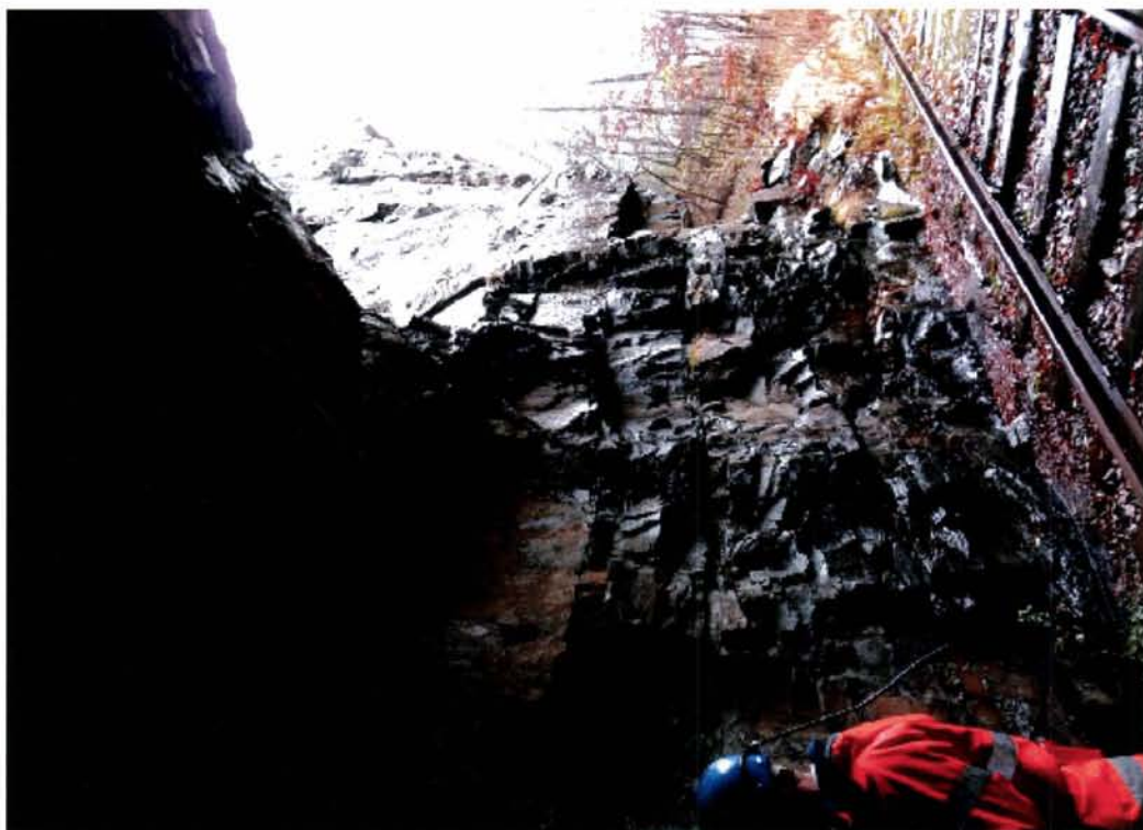
Km 16,280 11 Nov 2008 kl 11:40 Auestad tunnel S
