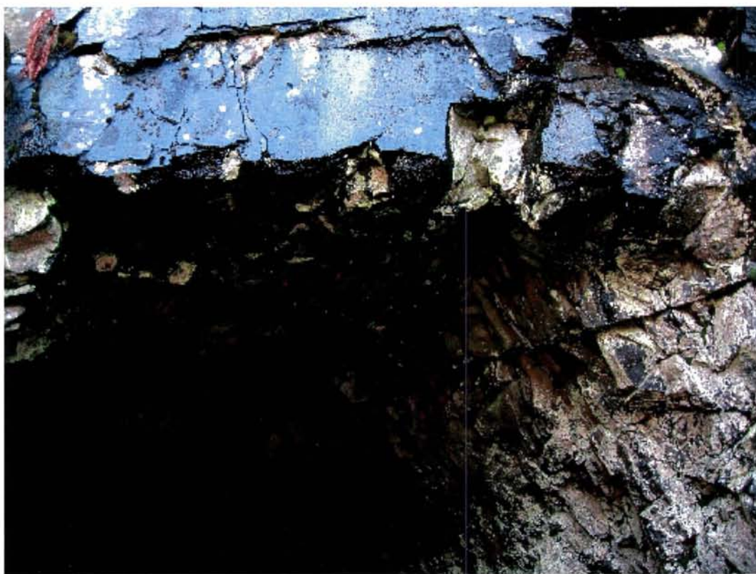
Km 12,960 12 Nov 2008 kl 11:44 Loga tunnel N
