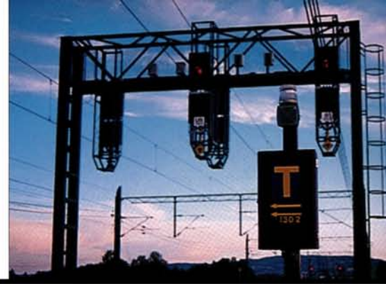
Signal gantry (bridge) on the Gardermobanen.
