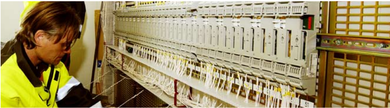
Part of safety installation. Photo: Jernbaneverket
