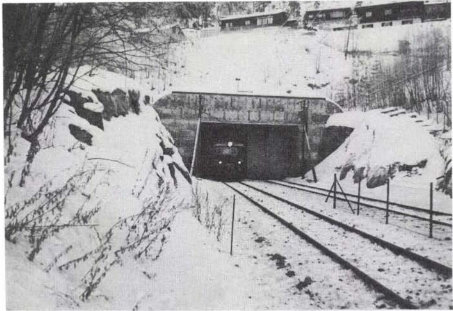
Fig. 72. Porten i Lieråsen tunnel.
