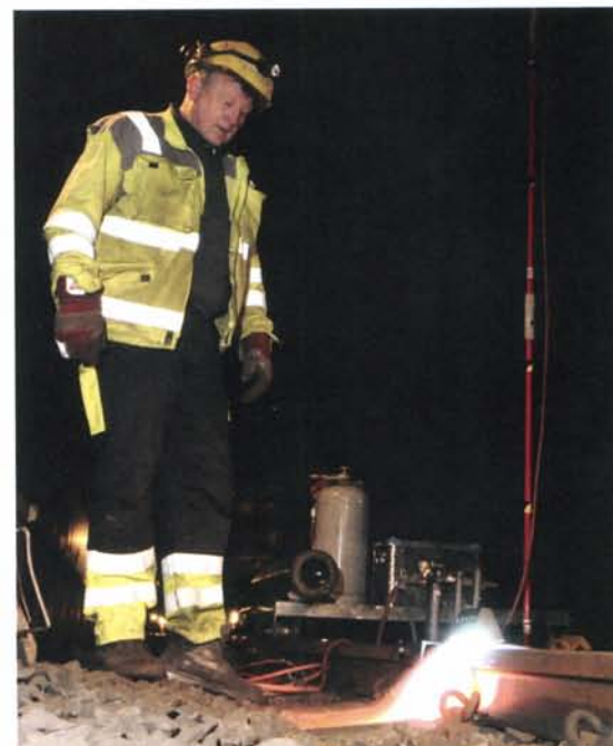
Rail renewal: New rails being installed in the Oslo tunnel.
