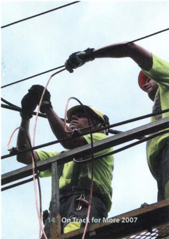
Sørland line: Catenary upgrading is necessary to supply sufficient electricity for train operations.
