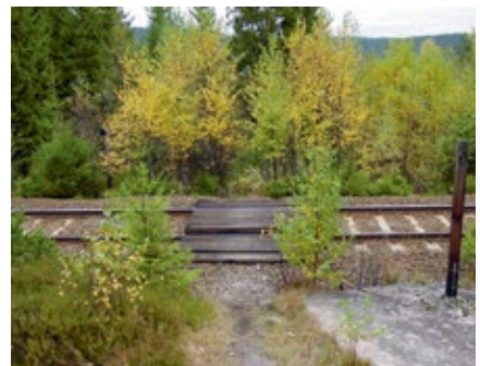
Usikret planovergang / Ungated level crossing
