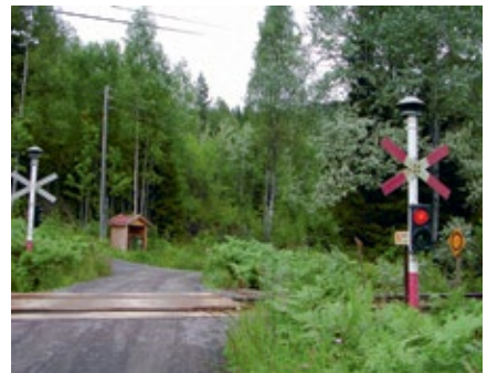
Veisignalanlegg / Warning lights
