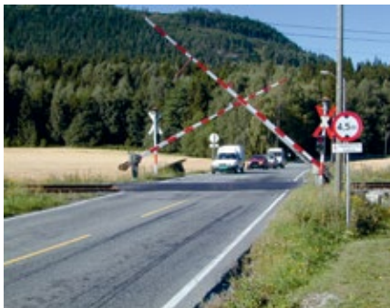
Helbomanlegg / Full barrier
