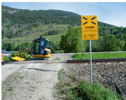
Grind/Level crossing gate
