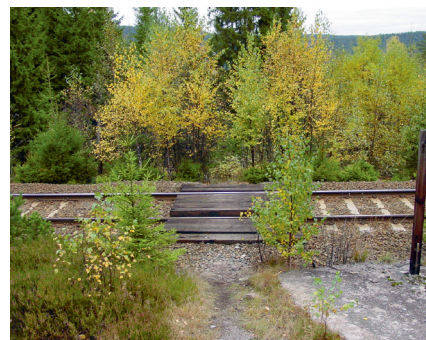
Usikret planovergang/Ungated level crossing
