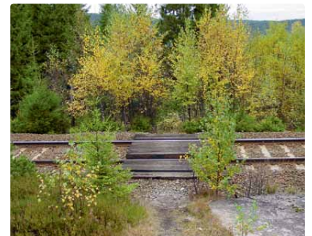
Usikret planovergang/Ungated level crossing
